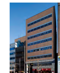
JRE Kayabacho 2Chome Building
