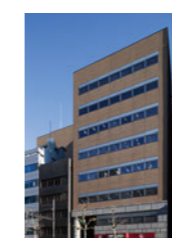
JRE Kayabacho 2Chome Building
